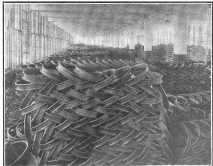
Stockroom of the Standard Welding Company, Cleveland, O., showing the method of storing the rims in stock
